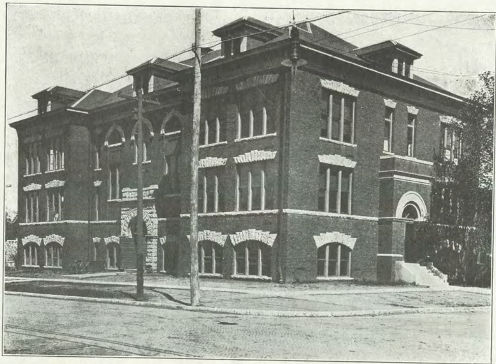
MANUAL TRAINING BUILDING
