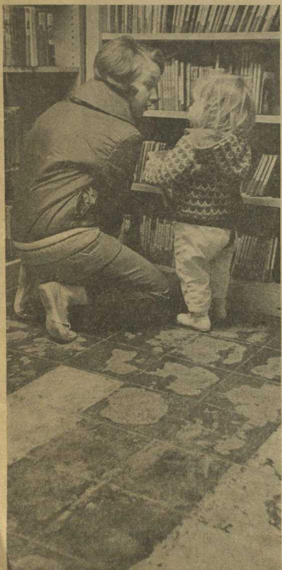
Floor damage from water . . .
